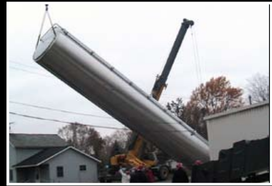
A series of photos show the delivery and installation of a new silo that can hold up to 600,000 pounds of milk.
