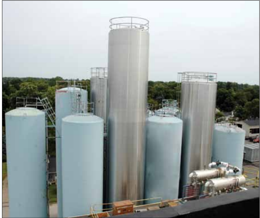
New raw milk storage silos have increased Ovid's raw milk storage capacity by 600,000 pounds.
