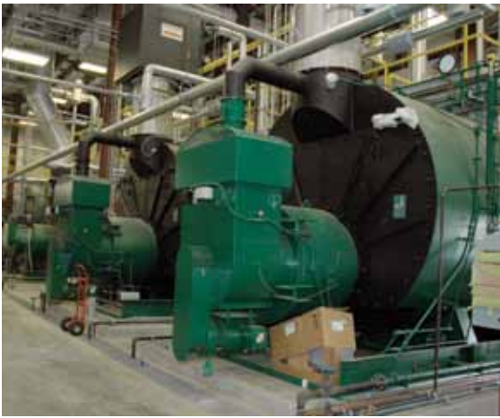
Two new boilers were installed and two existing boilers were relocated into the new boiler room. The additional boilers increase the plant's steam capacity to meet the utility demands of the new plant equipment. The boilers are used to supply high pressure steam to the operation.
