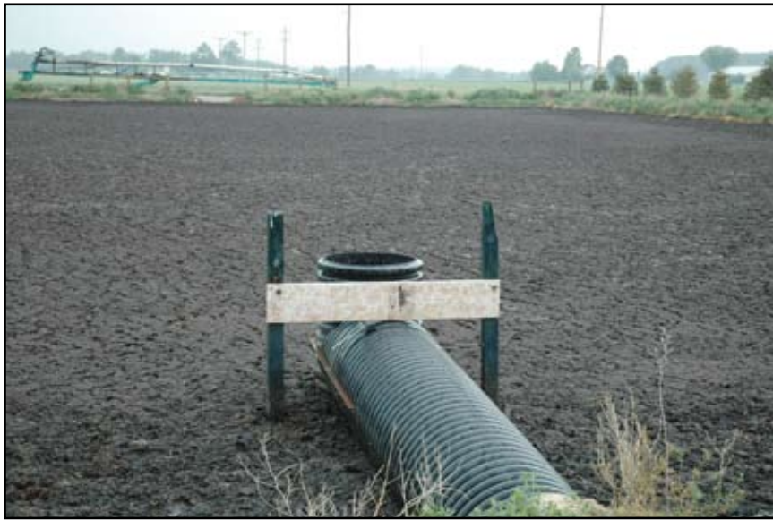
(pictured left) The “T” outlet allows the water to flow through, leaving the organic matter behind in the lagoon. (top) Tony Jandernoa, St. Johns, Mich., installed one of the first sand lane for manure separation in Michigan.
