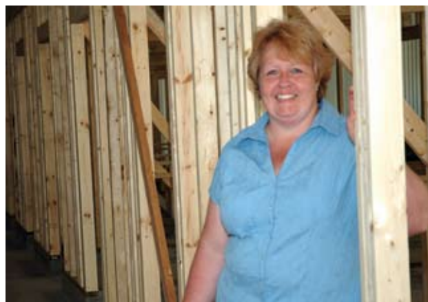
Wendy Powers stands in the doorway in one of the soon-to-be-completed chambers at the Animal Air Quality Research Facility. Open house participants will get a chance to see how the chambers help measure emissions for various animal species during the Oct. 13 event.
